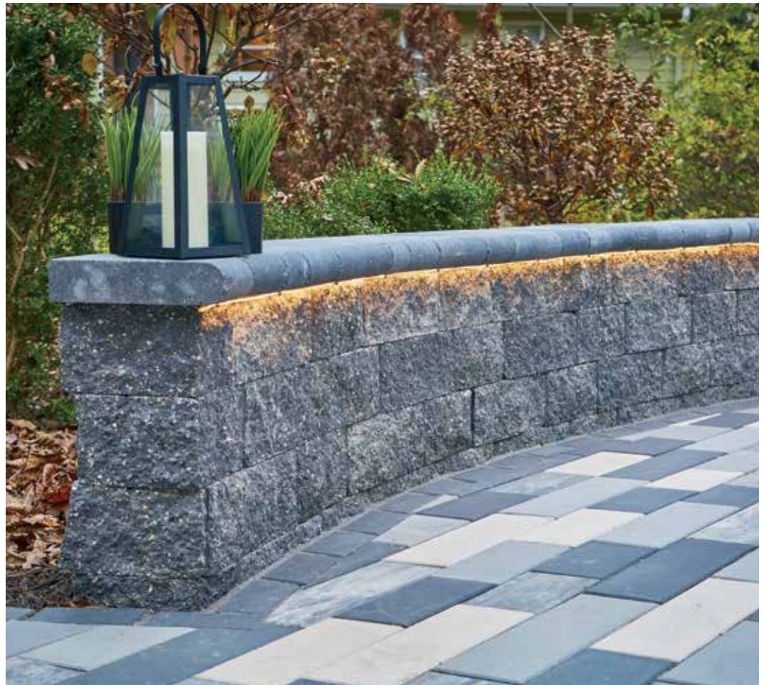
Tribute Retaining Wall System – GRAPHITE color (with Influence Pavers – DREAM, REFLECTION, VISION & MAJESTIC colors, and Crest Bullnose Pavers as seat wall caps – REFLECTION color)
