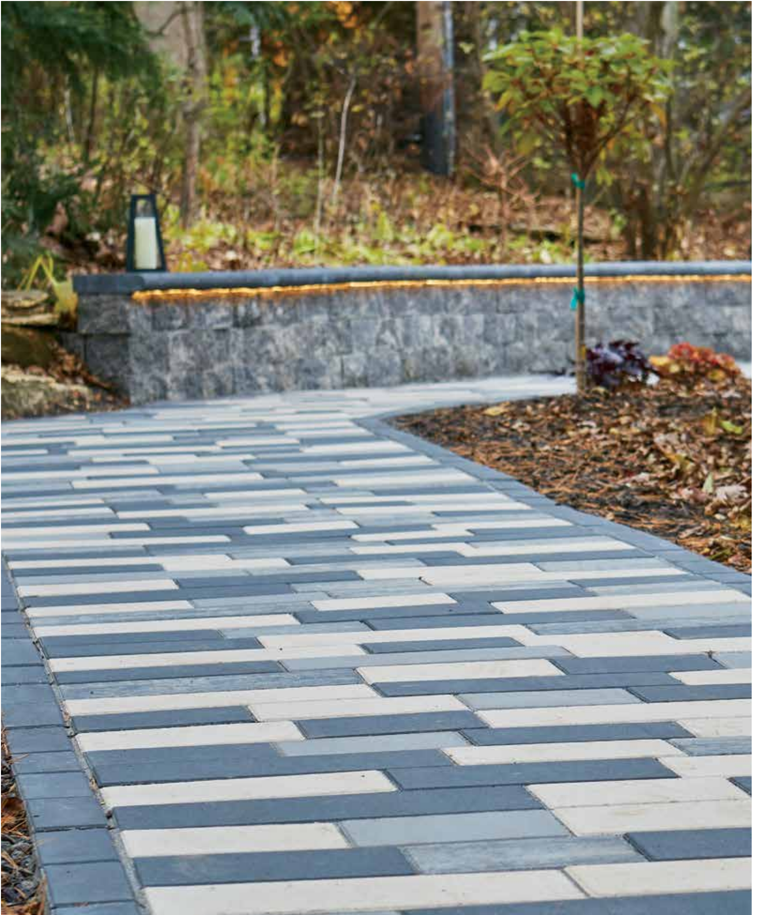
Influence Pavers – DREAM, REFLECTION, VISION and MAJESTIC colors (with Elements Paving Stones border – REFLECTION color)
